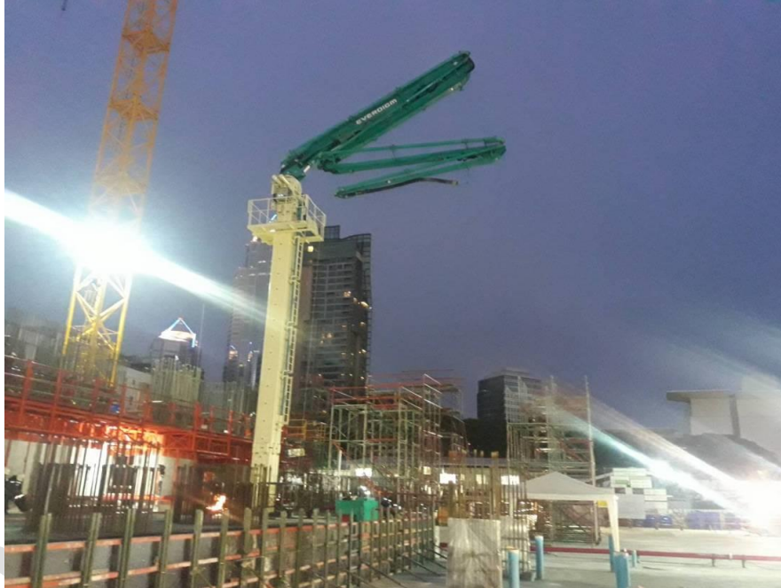
CONCRETE PLACING BOOM
